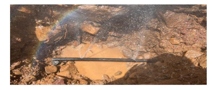
Bedding and compaction previously used also contributes to leaks as seen below.
