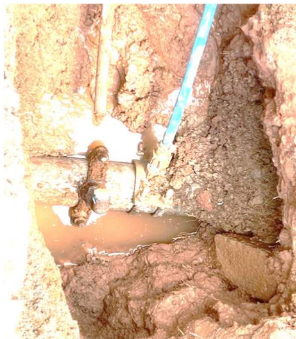
Repaired with correct installation
